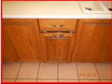
Faucet and Supply Lines:
