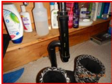
Faucet and Supply Lines:
